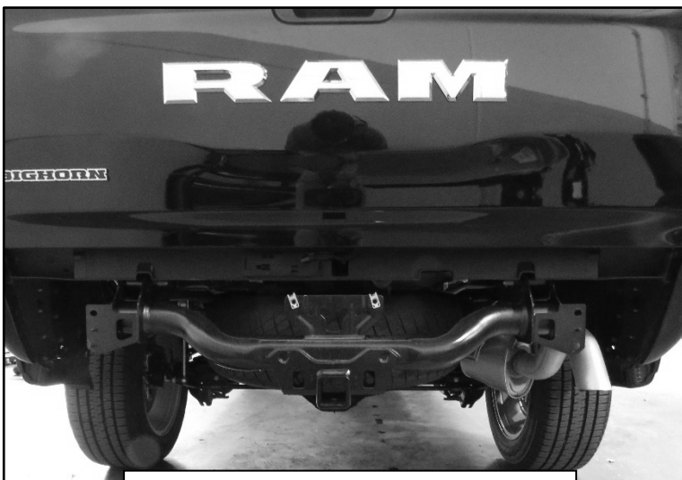
(Fig 5) Bumper completely removed
