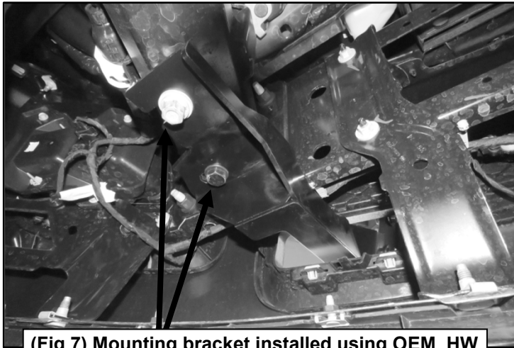
(Fig 7) Mounting bracket installed using OEM HW and supplied HW
