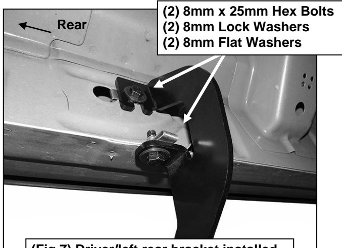
(Fig 7) Driver/left rear bracket installed
