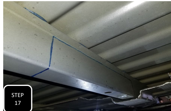
Step 17 Measure and mark a line 15 inches out from the heat shield that you just cut out then draw a cut line up both sides and along the top .
