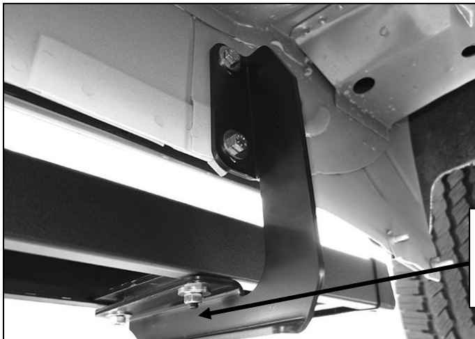
(Fig 10) Driver/left front mounting Bracket installed
