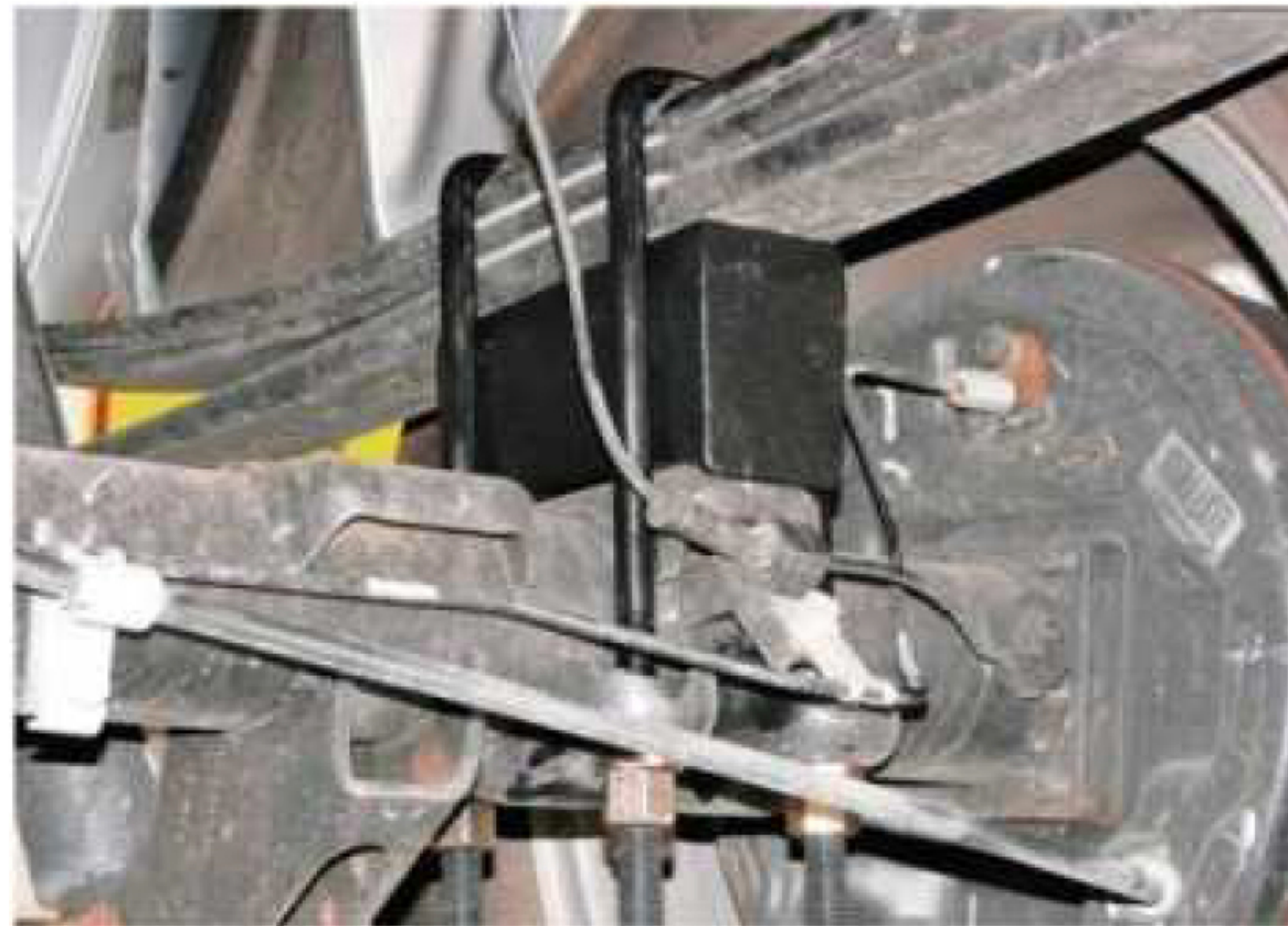
The installation photo for reference
