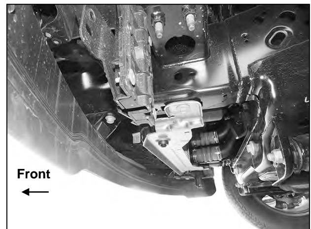
(Fig 2) Active air dam removed
