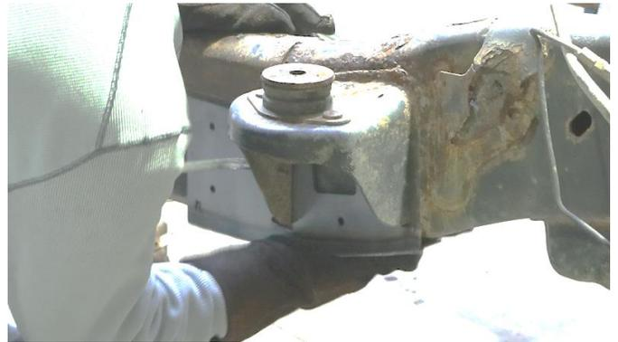
Following proper welding procedures, tack weld your front frame section into place before welding the part on fully. Weld 100% around all edges.
